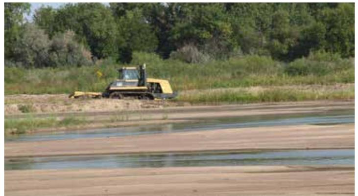
*During low flows in the Platte River during October, sandbars at Rowe were disked to clear unwanted vegetation. This annual maintenance of the wide, braided channel assures suitable habitat conditions for roosting cranes in the spring.*
